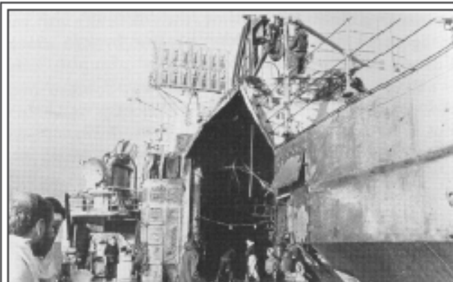
Figure 5: HMS Glamorgan shortly after being hit by land-launched Exocet. The hole in the galley deckhead has been covered with plywood sheets
